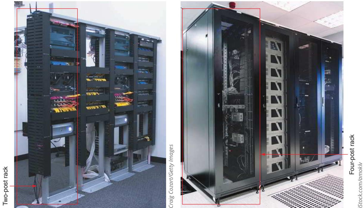
**Figure 2-11** Open two-post racks and enclosed four-post racks
