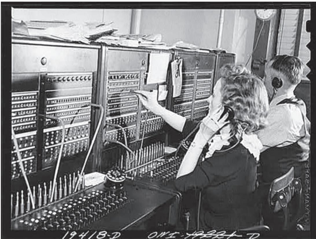
**Figure 7-1** A mid-twentieth century telephone switchboard
