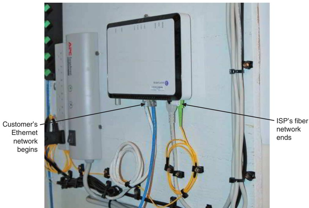
**Figure 2-3** Demarc for Internet service to a campus network; this demarc is located inside a small data room and connects the incoming fiber signal from the ISP with the campus's Ethernet network
