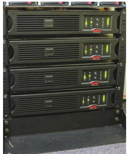
**Figure 12-27** Online UPSs installed on a rack
