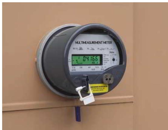
**Figure 10-28** A single-use, plastic security seal
