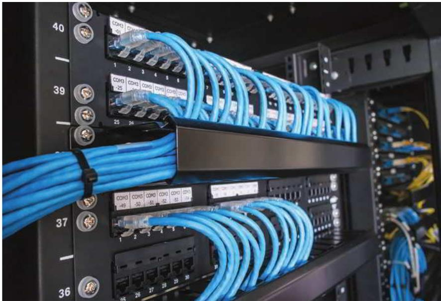
**Figure 2-5** Patch panel on rack
