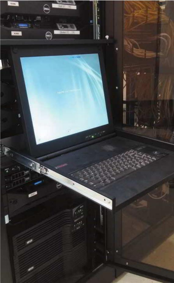
**Figure 2-13** Here, a single console uses five KVM switches to access and configure multiple devices in a row of racks
