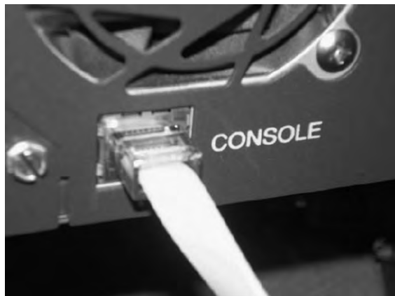
Figure 11.2 Console Port on a Cisco Switch with Console Cable Attached
