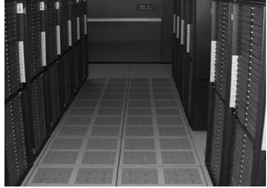
FIGURE 4-28 One aisle showing a number of racks of a very large computational cluster. Notice that the floor consists of perforated tiles, which provide cooling from beneath the raised floor. Note that the nodes in the rack take cooling in from the front and export warm air out of the back. Therefore, in most computer rooms, you will notice alternating cool and hot aisles, where each aisle consists of either fronts (cool aisle; perforated tiles) of two sets of racks, or backs (warm aisle; no perforated tiles) of two sets of racks.
